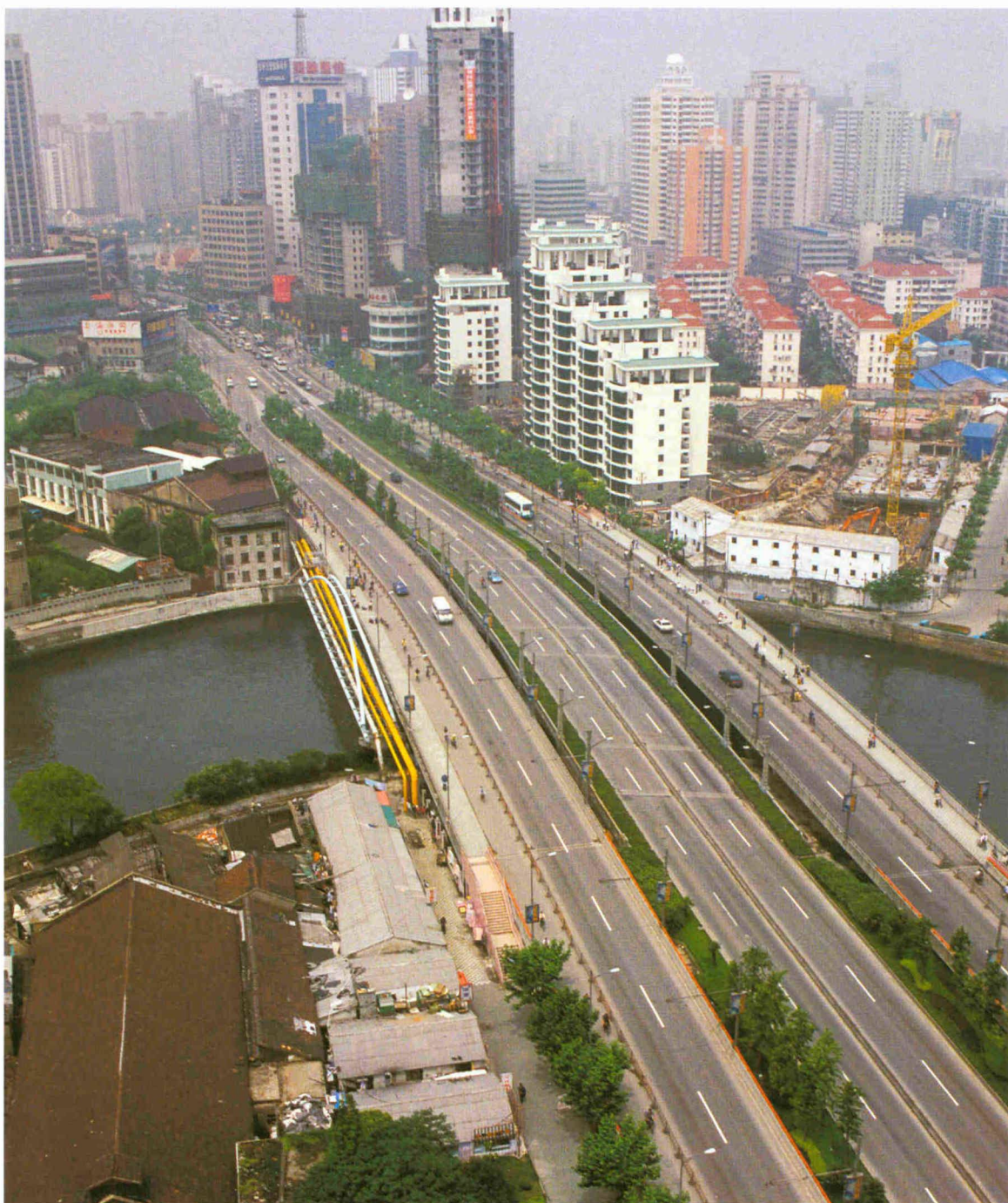
长寿路桥 Changshou Road Bridge
