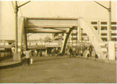
昌化路桥旧貌 The Old Site of Chang Hua Bridge
