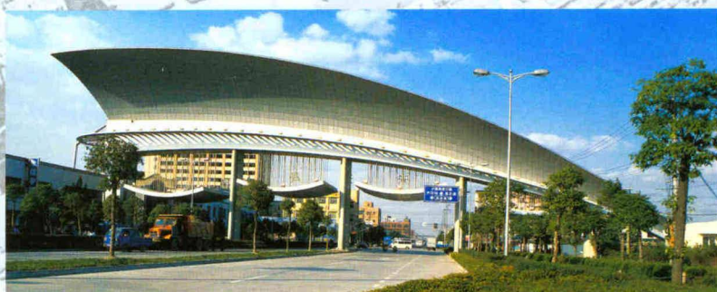
上海西北综合物流园区 Shanghai Northwest Comprehensive Logistics Park
