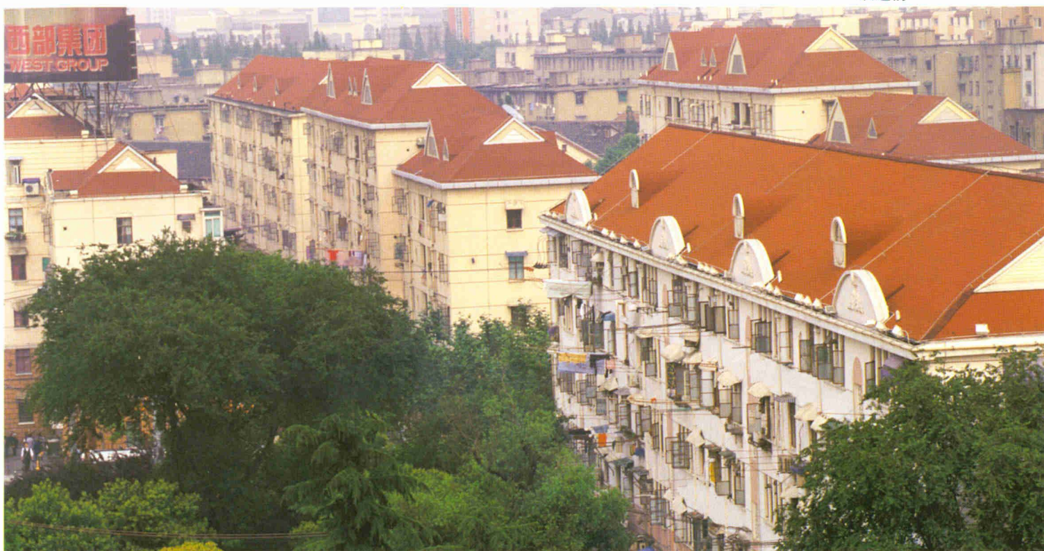
改造后 After Reconstruction
