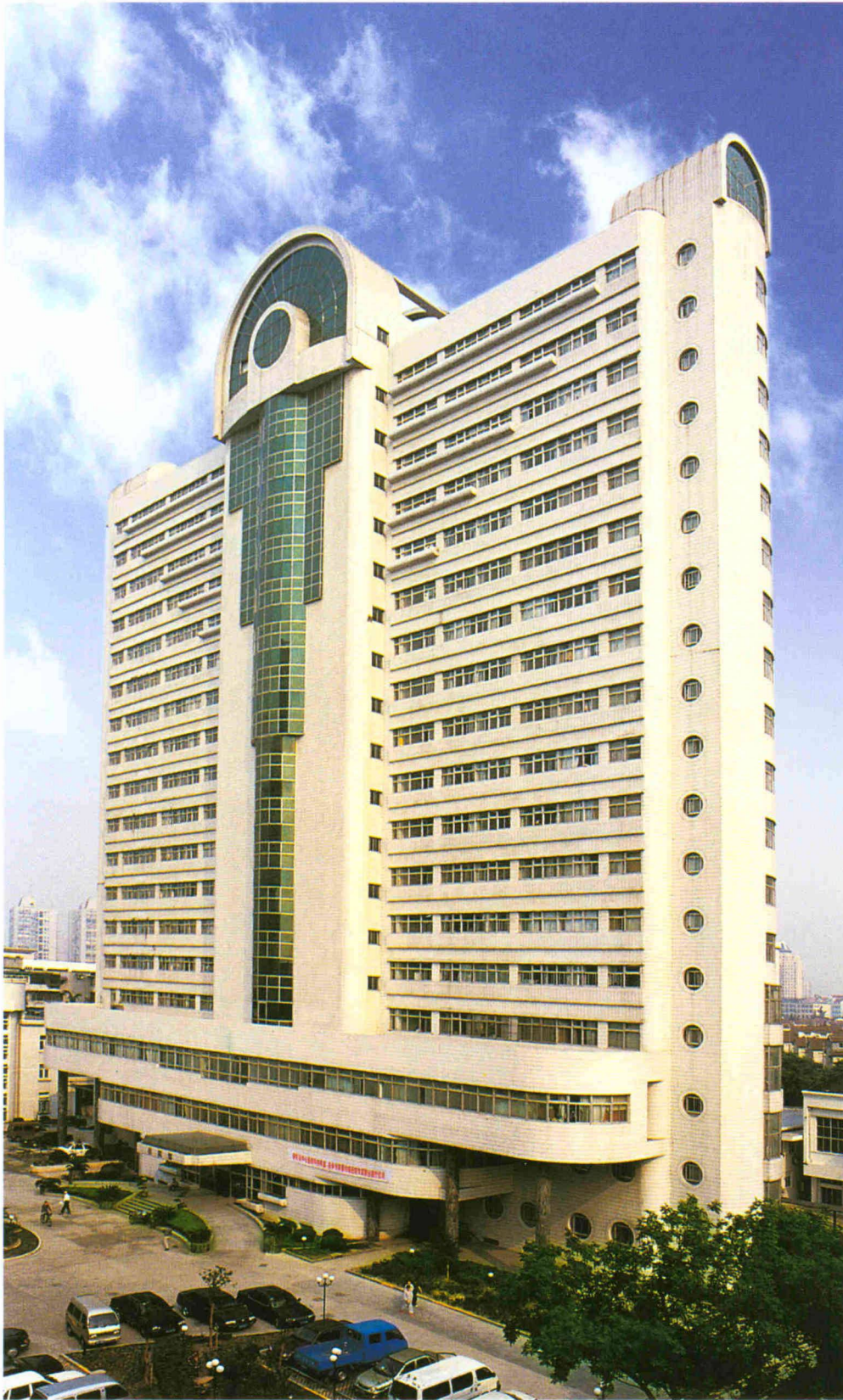
普陀区中心医院新建病房大楼 Putuo Center Hospital and its newly built ward
