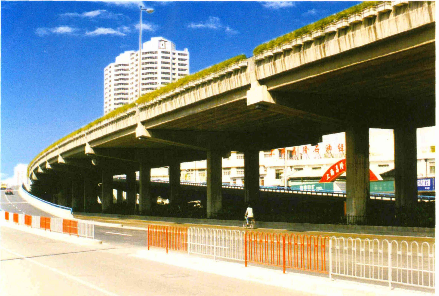
内环线金沙江路匝道 The Jing Sha Jiang Lu Ring Road of The Elevated Inner Ring Road
