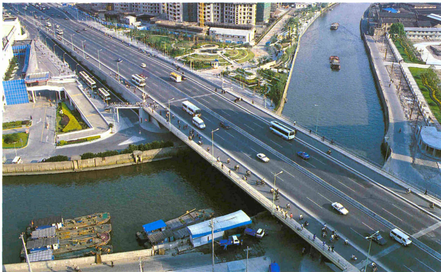
拓宽后的武宁路桥 Renovation Project of Wuning Road Bridge
