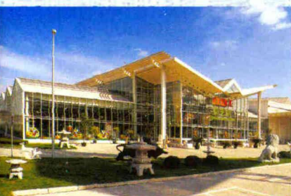
上海华德美超市有限公司(欧倍德普陀店) Shanghai Homeworld Supermarket Company Limited (OBI Putuo Shop)
