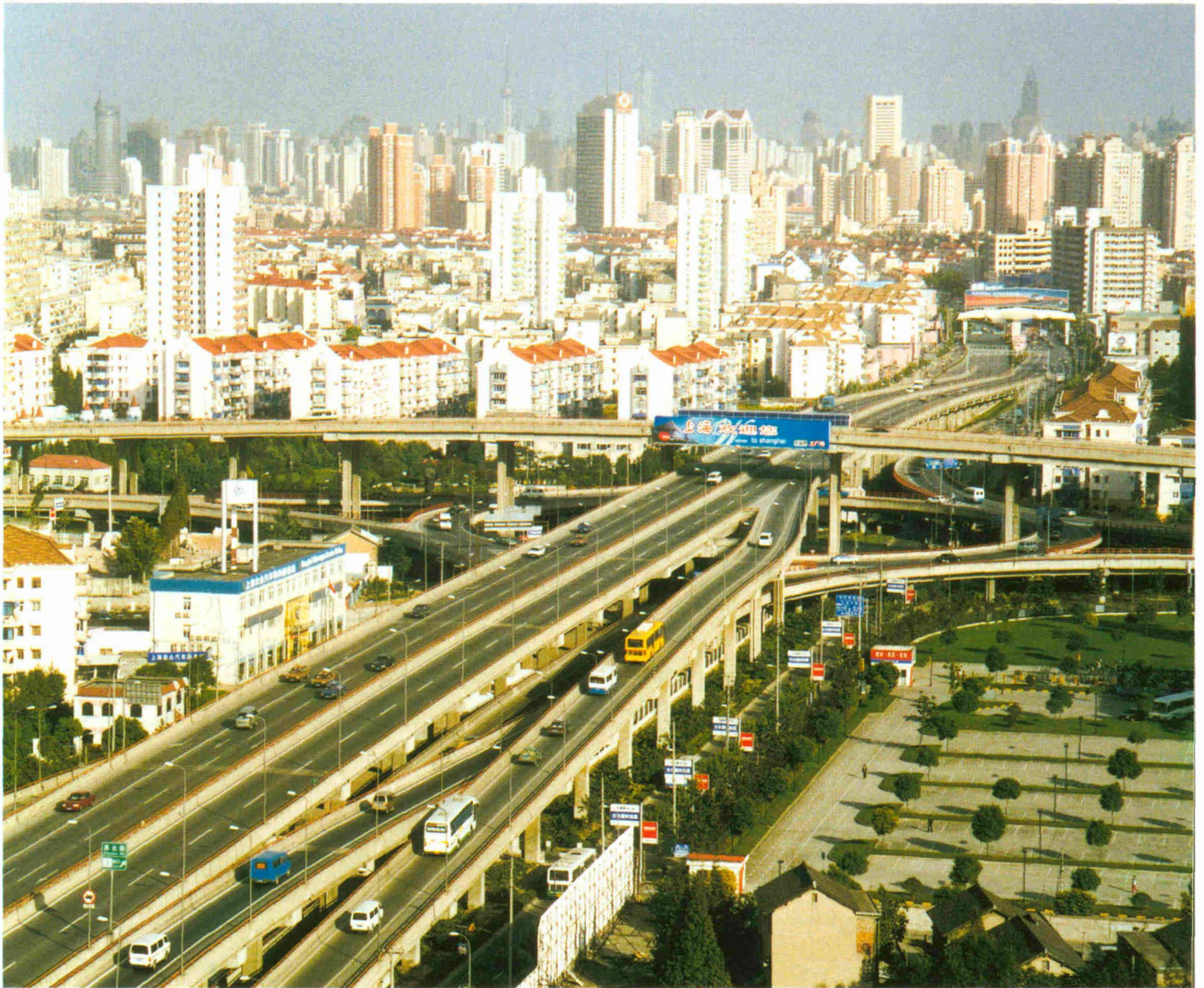
沪宁高速公路入城段 The Putuo Section of Hu-ning Expressway
