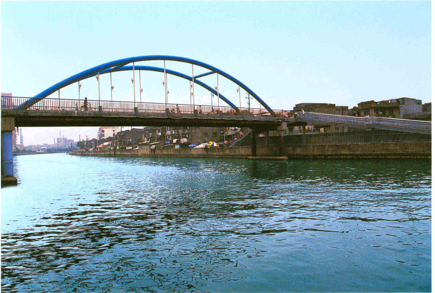
强家角人行桥 Qiangjiajiao Pedestrians' Overpass
