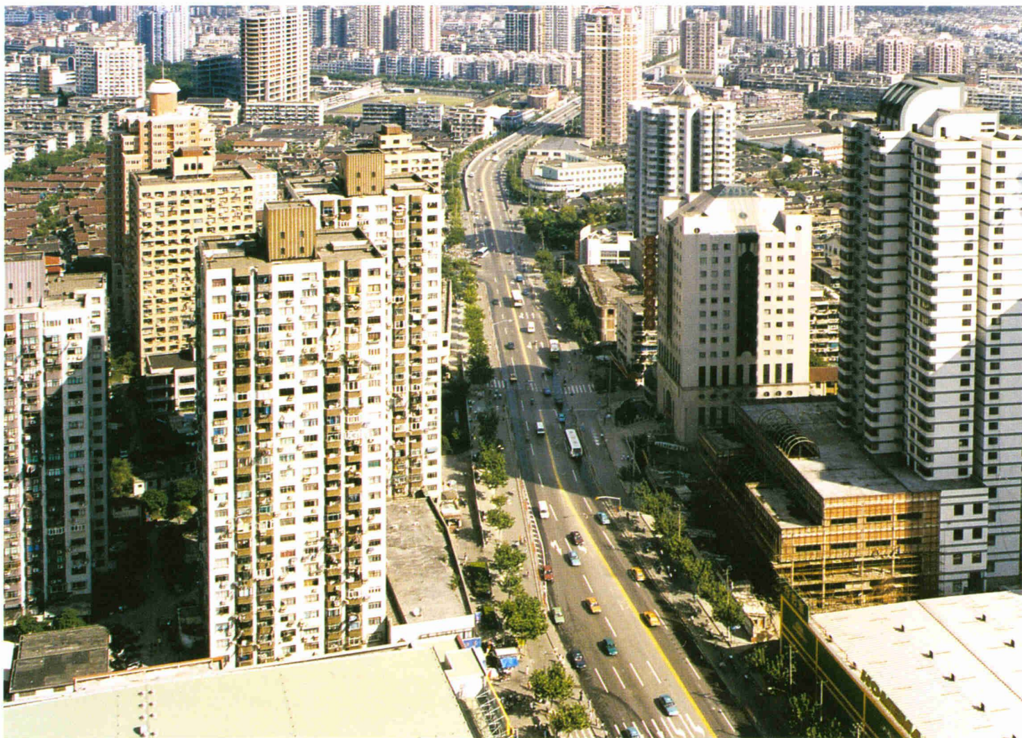
改造后的朱家湾地区 Zhu Jia Wan Area Which After Reconstruction
