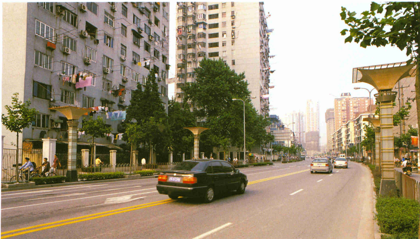
辟通后的宁夏路 Ningxia Road after Opening
