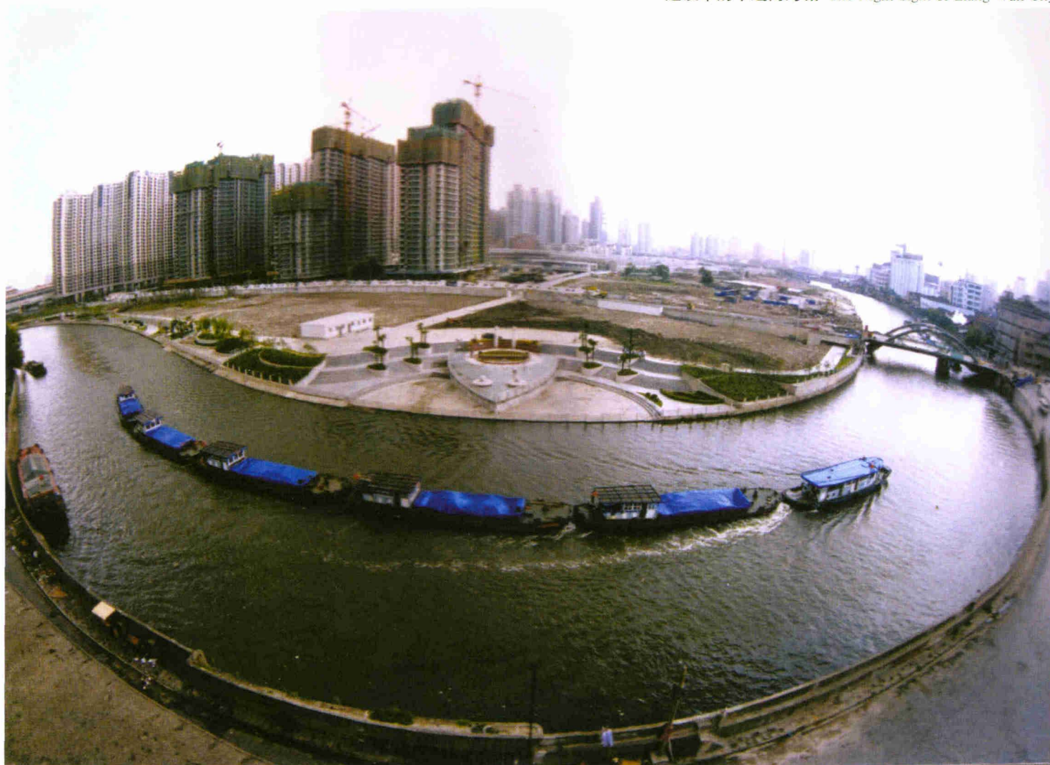
建设中的中远两湾城 COSCO Liang Wan City Which is Unnder Construction
