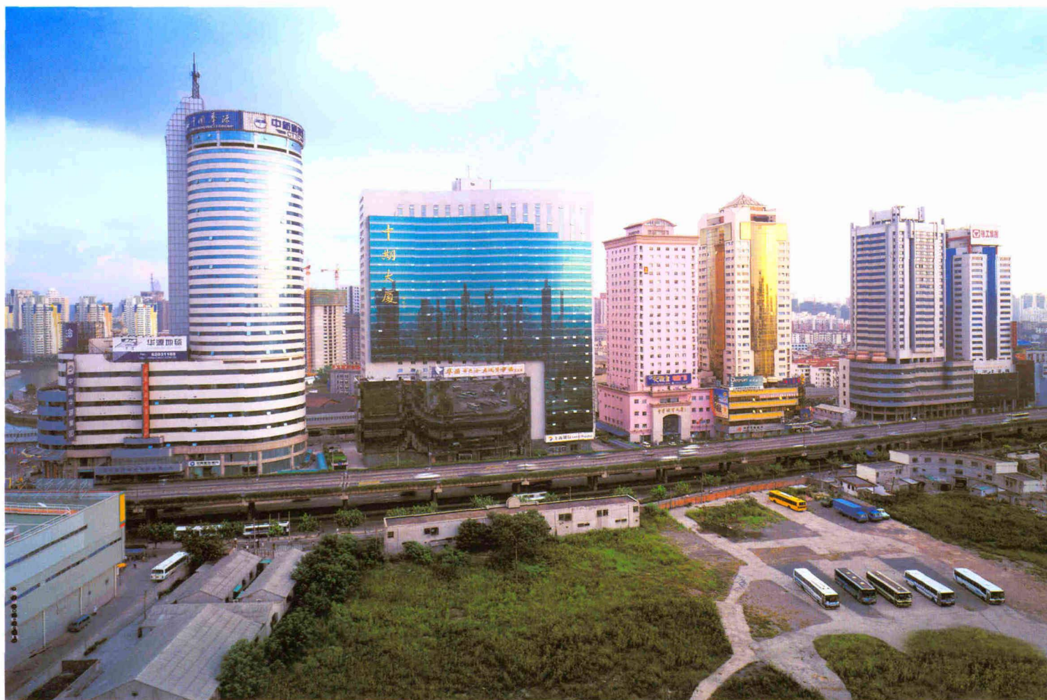
中山北路物贸街 A Goods and Material Exchange Street on Zhongshan North Road
