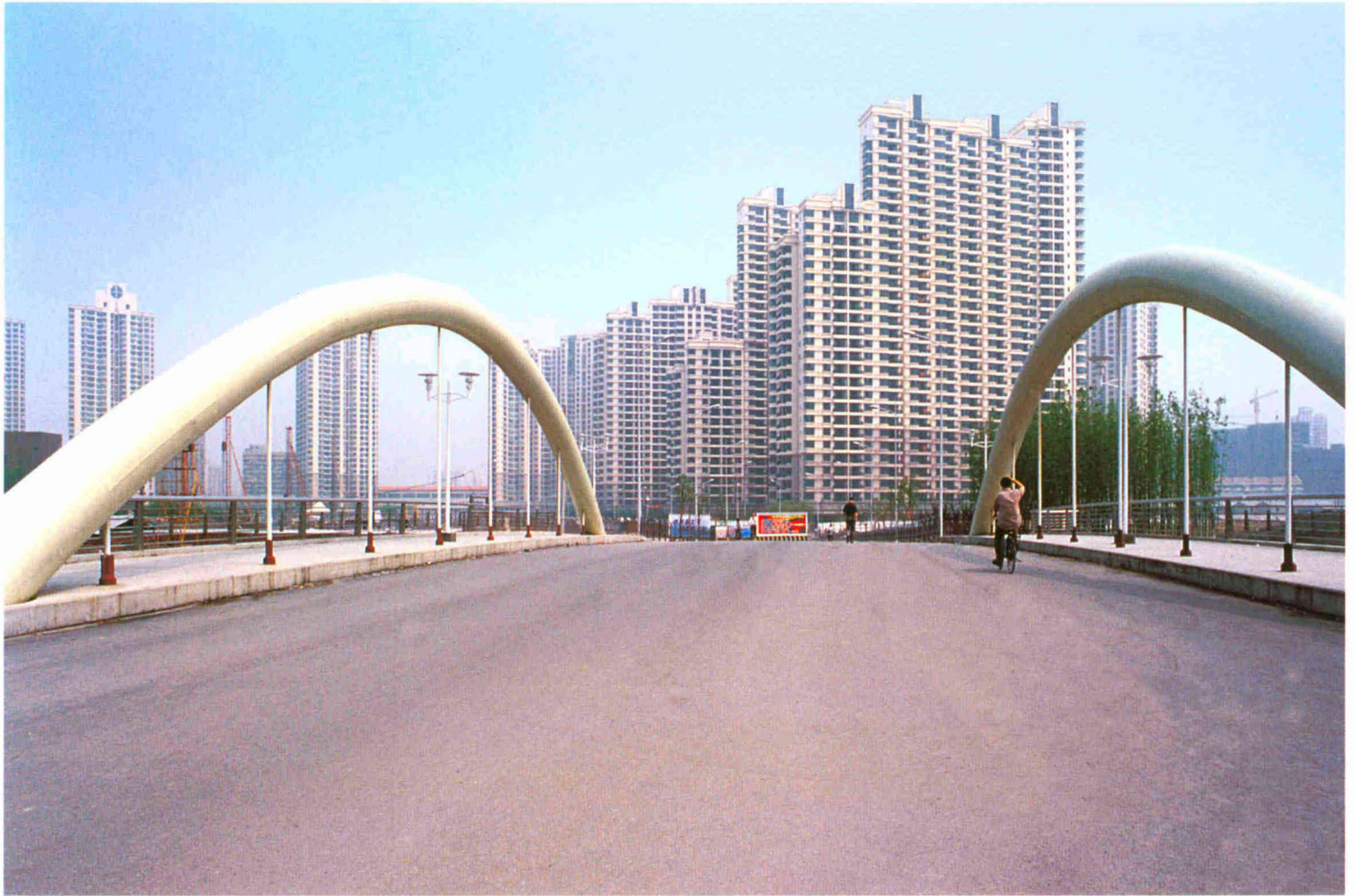
新建的昌化路桥 Rebuilding Project of Changhua Road Bridge
