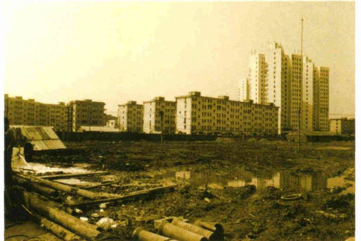
普陀区区级机关综合办公楼原址 The Old Site of The Comprehensive Official Building of Putuo District
