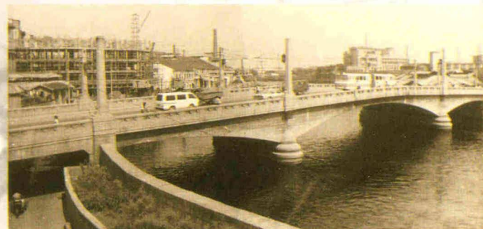
长寿路桥旧貌 The Old Chang Shou Road Bridge
