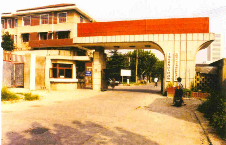
原区级机关大院 The Old Official Building of Putuo District
