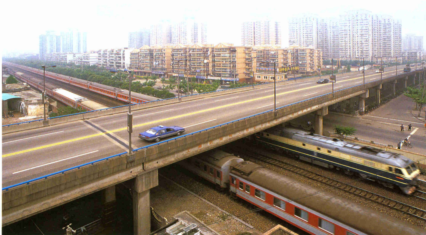
光新路（铁路）立交桥 Guangxin Road (railway) Overpass
